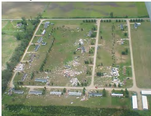
Foster Trailer Park Tornado Damage
