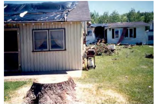
Tornado Damage, Forest County
