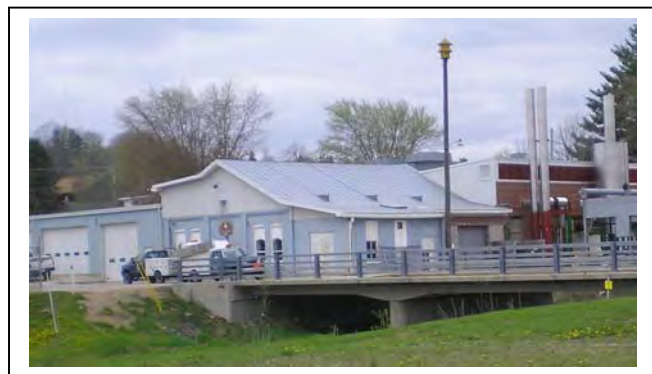
Municipal Garage also contains electric generating equipment
