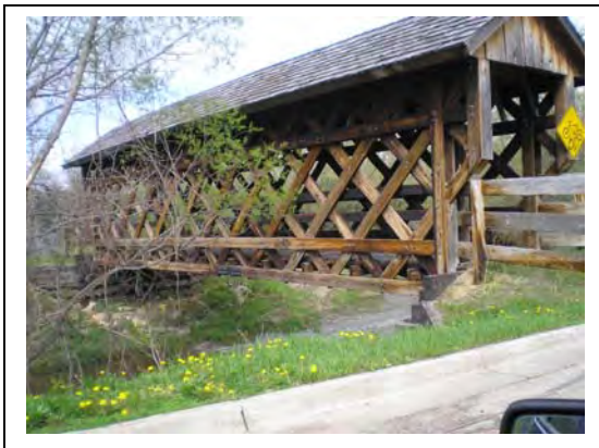
This bridge carries the Omaha Trail over the Baraboo River
