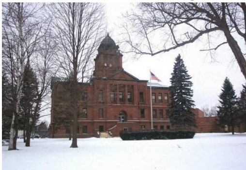
County Courthouse, Antigo.
