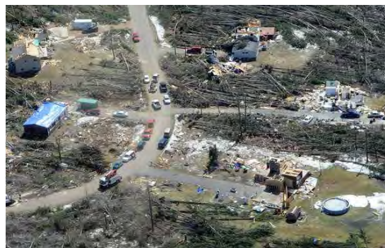
2011 Tornado Damage, Merrill
