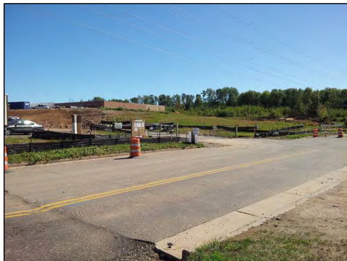
New Walmart Under Construction
