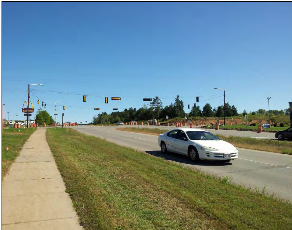
Existing Sidewalk along North Side of STH 64 / E. Main Street
