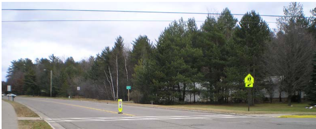
Well designed crosswalk – 1. high visibility painted crosswalk 2. appropriate sign 3. in-street paddle sign for extra emphasis.
