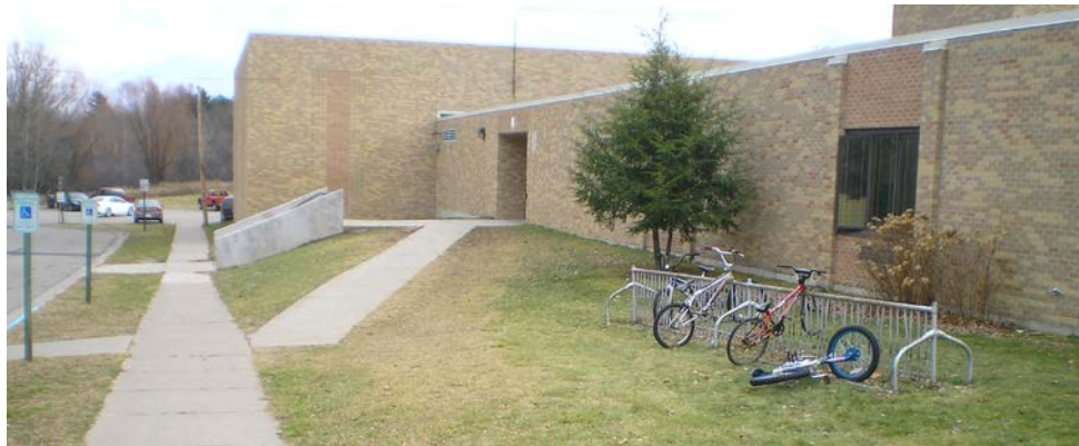
Bike racks prominently located at an entrance, but are not well used.
