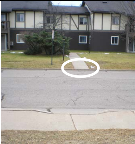
Acacia Ln, west of JWMS building
