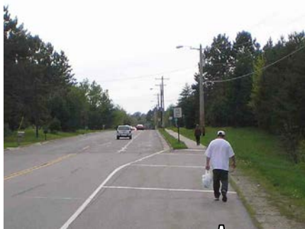
Picture taken at “ A ” E. Timber Dr bike lane
