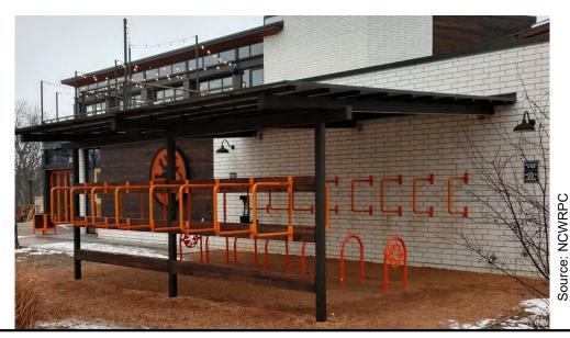
Wall racks maximize capacity. Ground racks are convenient to understand.
