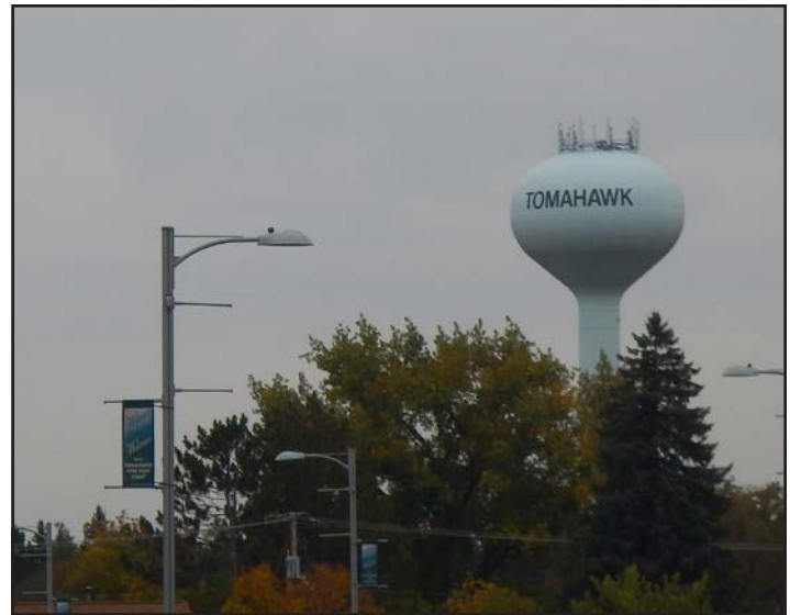
Tomahawk Water Tower
