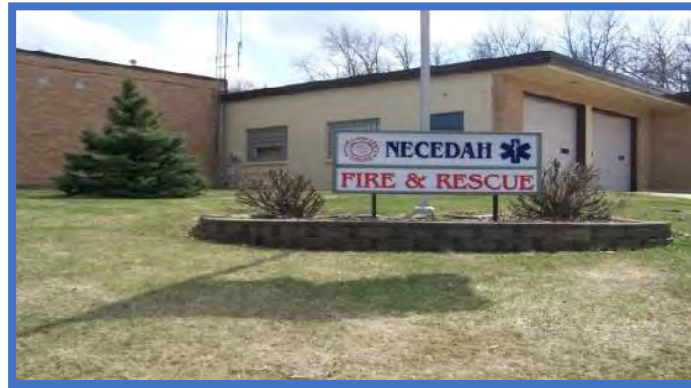
Necedah Fire Station
