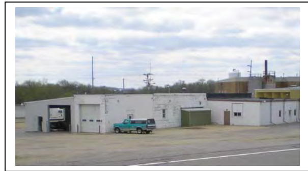
Town Hall & Garage
