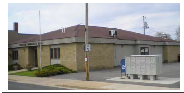
Village Hall & Community Center
