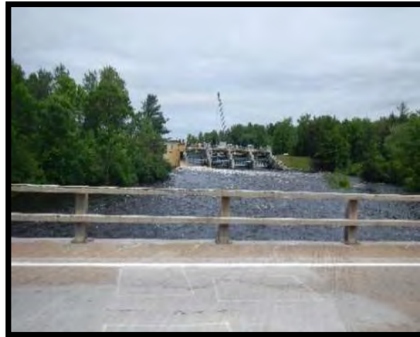
Dam in Northern Lincoln County
