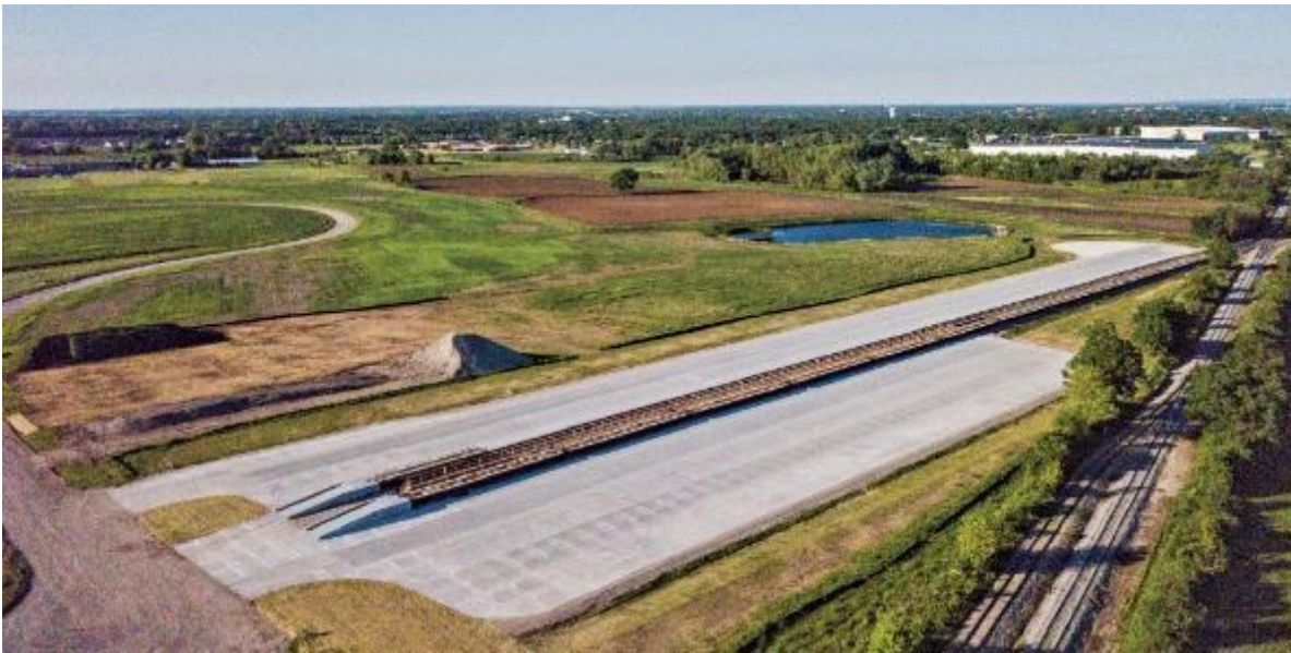
Figure 88 WSOR Oshkosh, WI Transload Facility
