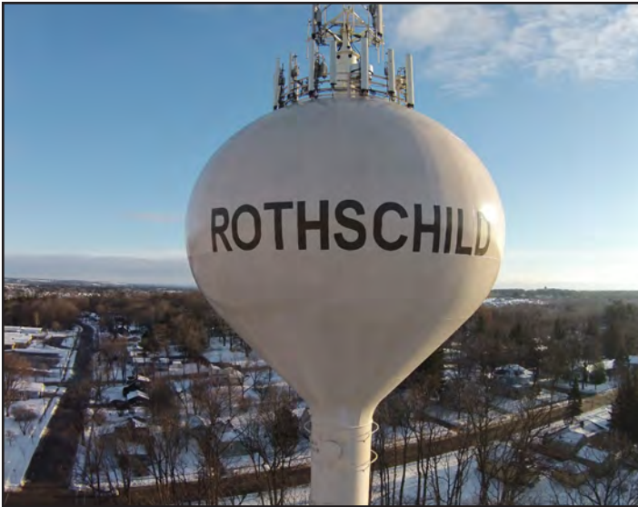
Water storage facilities include the watertower
