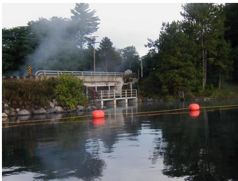
Rest Lake Dam. (WDNR)
