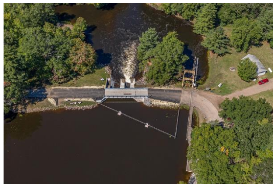
Rollaways Reservoir Dam & Boat Hoist (WVIC)
